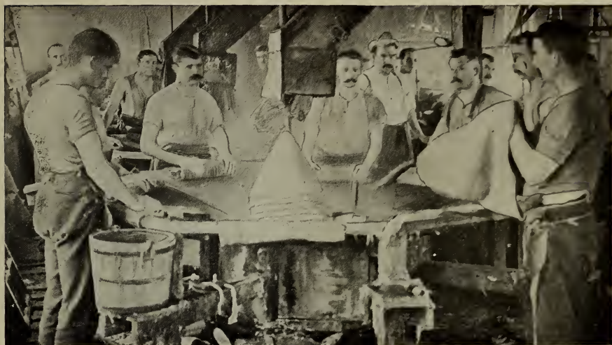
"SIZING" OR SHRINKING THE HATS
